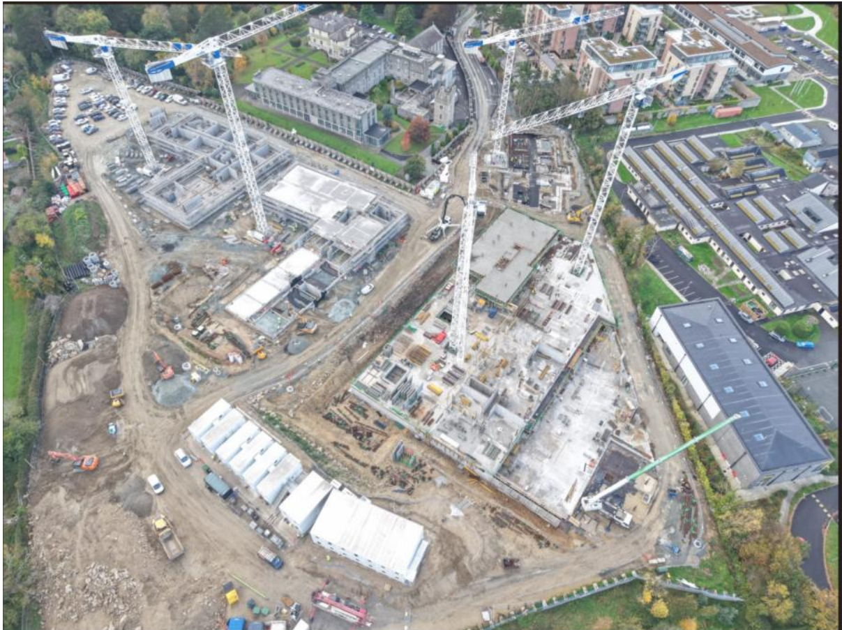
Figure 2 Image of wider site, with blocks A to D currently under construction
